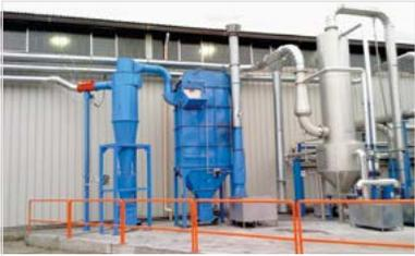
Steel dust extraction systems on rolling line - Atex
